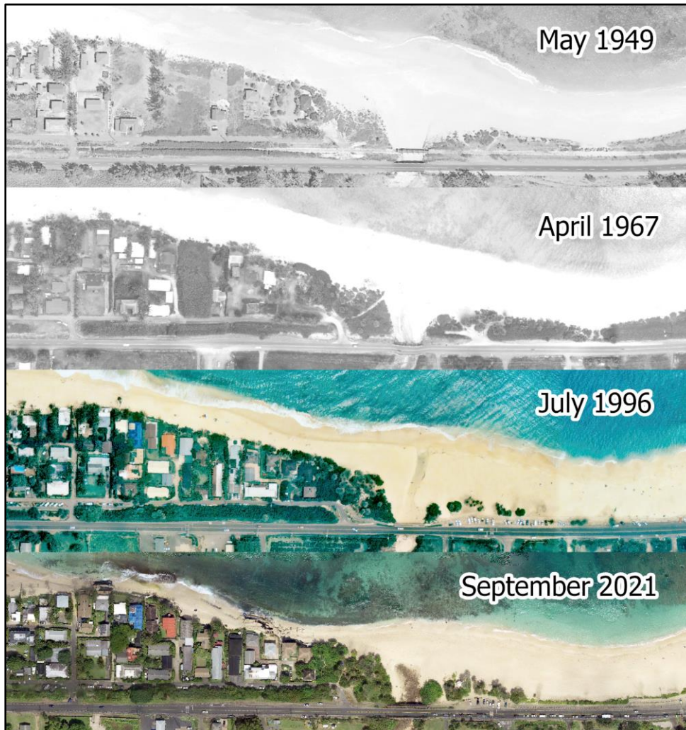
Figure 5. Erosion of Sunset Beach over time. (Source of Images: Climate Resilience Collaborative, 2022b. Figure compiled by Authors.) Though images depicted are taken at different times of the year, and beach widths on the North Shore of O’ahu vary depending on seasonality, there is documentation of chronic erosion occurring in this area, which can be seen in the changes in vegetation (Climate Resilience Collaborative, 2022a).
