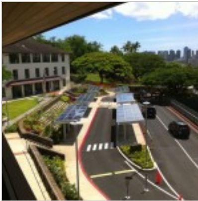
Punahou School, Omidyar K-1 Building, PV Panels Shading Drop Off Area
